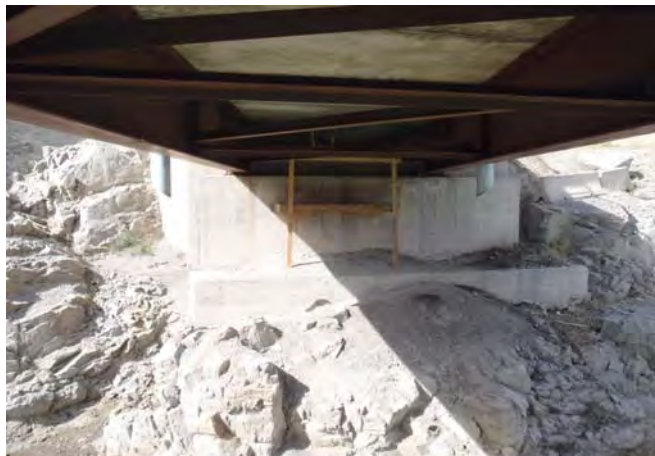
Figure 1-26: Woods end abutment.
