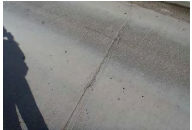
Figure 1-14: Typical deck panel joint condition.
