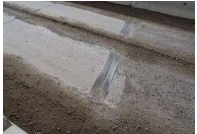
Figure 1-8: Woods end abutment joint.
