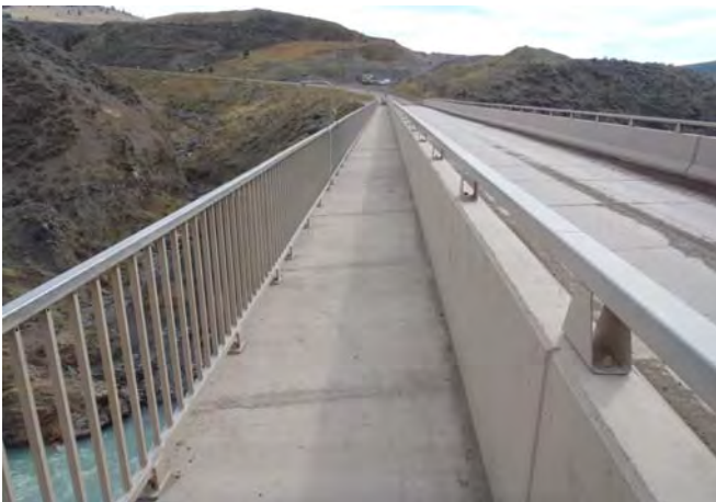
Figure 1-9: Upstream sidewalk condition.
