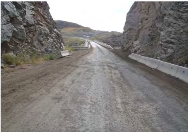
Figure 1-3: Looking towards camp end.
