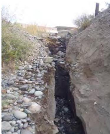
Figure 1-25: Drainage channel adjacent to camp end abutment.
