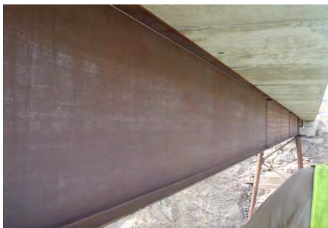
Figure 1-21: Typical girder condition, span 2 upstream shown.
